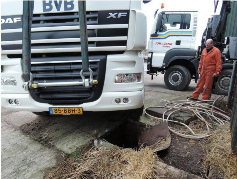
Hoisting with a crane
