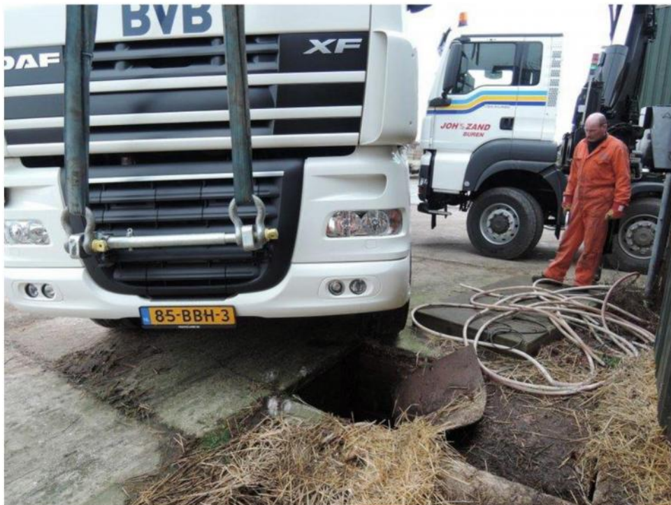
Lifting with beams and winch eyes
